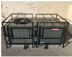
Two cages can be combined together to accommodate larger condensers and package units.
